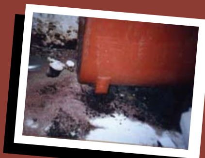
Corroded Leg
